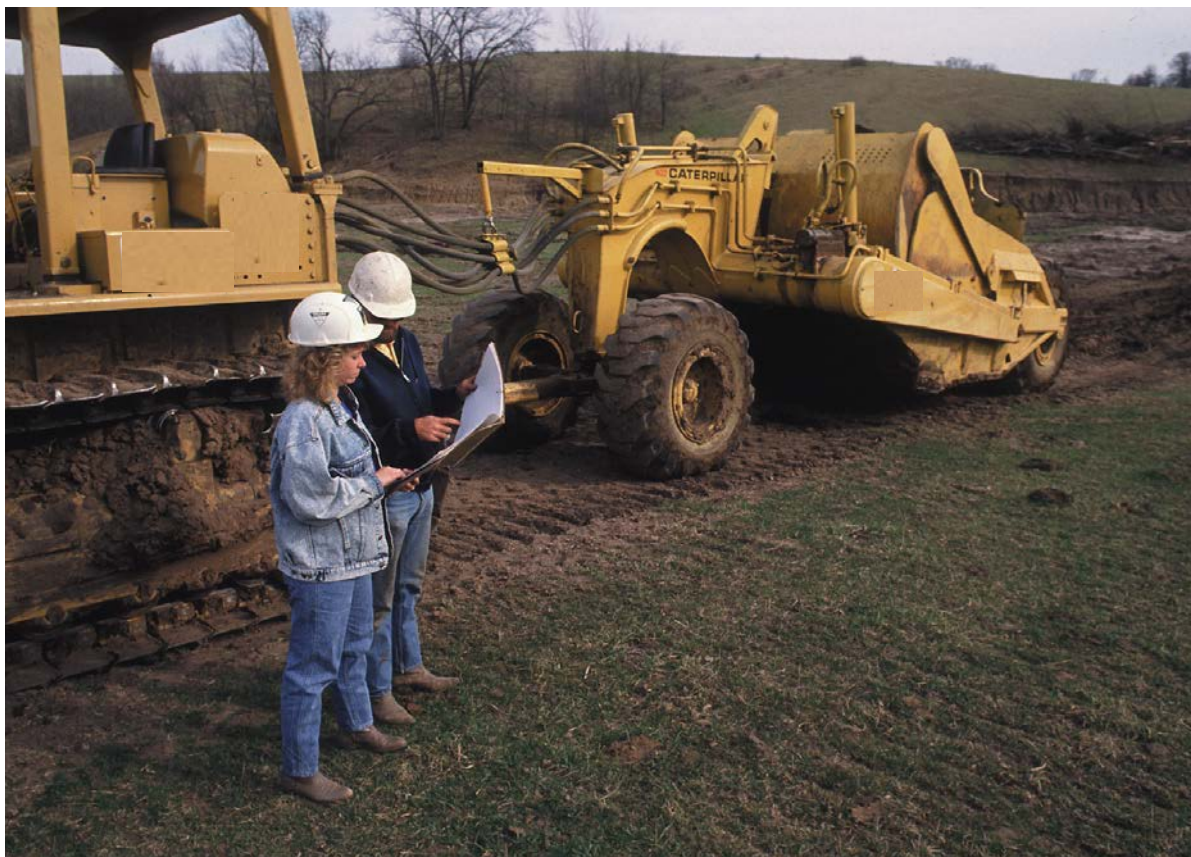
Figure 600-C10: Conservationist and contractor reviewing practice design in the field
