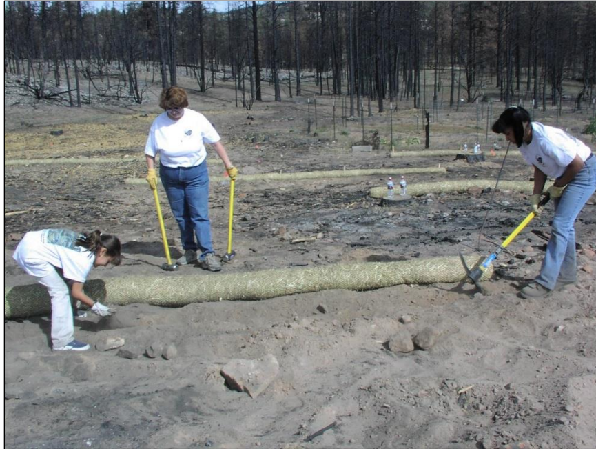
Figure 7-17. Volunteers install fiber rolls (also called wattles) on burned area prior to Critical Area Planting (342) to control erosion. Photo: USDA NRCS.
