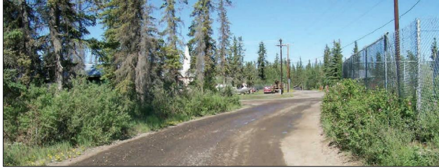
Figure 7-19. Water can provide temporary dust control on unpaved roads and surfaces. Photo: USDA NRCS. 130
