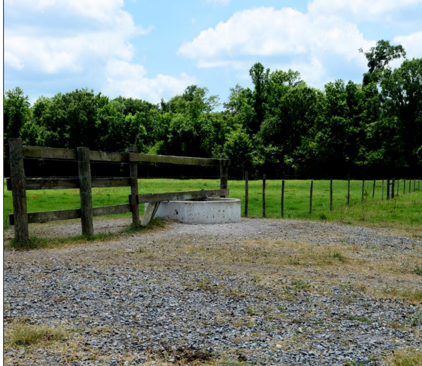
Figure 7-32. Heavy use area that has been armored with a surface of aggregates, Thibodeaux, Louisiana. Photo: Stephen Kirkpatrick, USDA NRCS.
