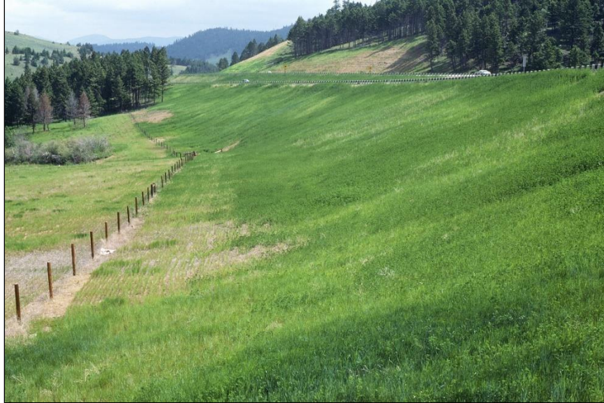
Figure 7-16. Herbaceous cover used to stabilize a roadside slope. Photo: USDA NRCS Montana.
