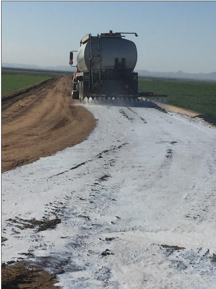
Figure 7-20. Commercial polymer being applied to farm road. Photo: Andrew Faison, USDA NRCS, Avondale Arizona.
