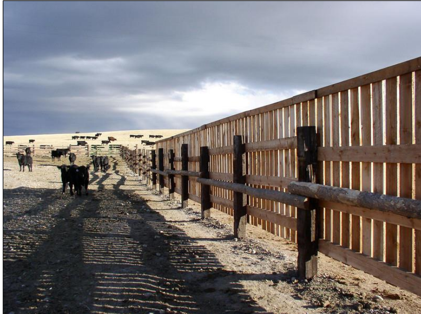
Figure 6-24. Where tree planting isn't possible, consider artificial windbreaks. This fabricated windbreak shelters livestock and protects the heavy use area from wind erosion. Photo: USDA NRCS, Gallatin County, Montana, 2007.
